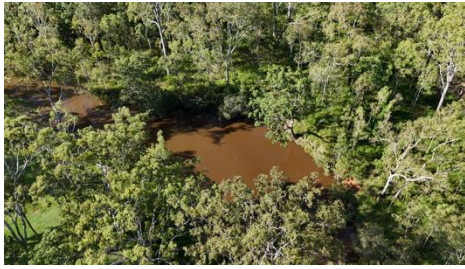
Turbidity in Yellori Creek from switching station runoff from rain event January 2024
