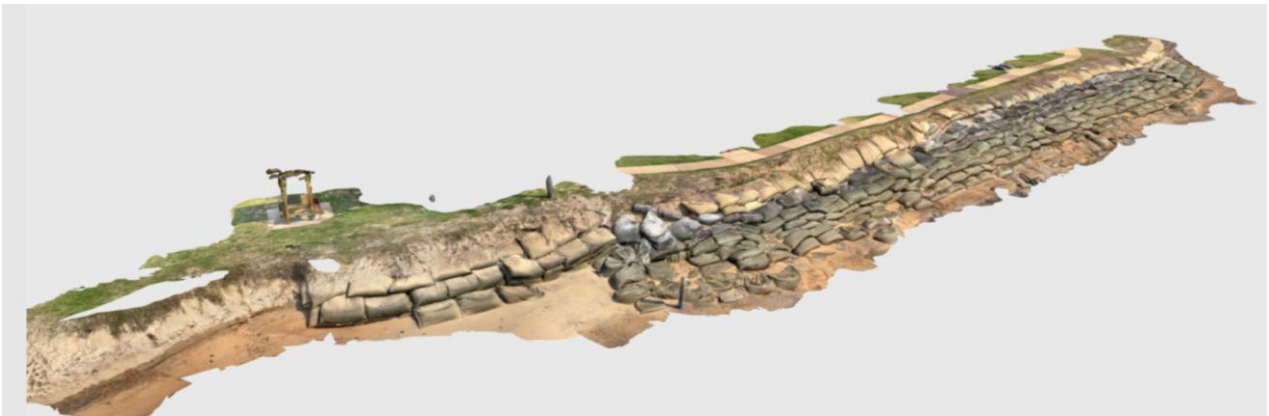
Figure 4-7 GSC Seawall Structure
