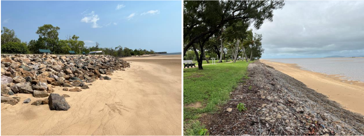
Figure 4-6 Left: Taylors Beach Rock Seawall. Right: Gabion Basket Seawall.
