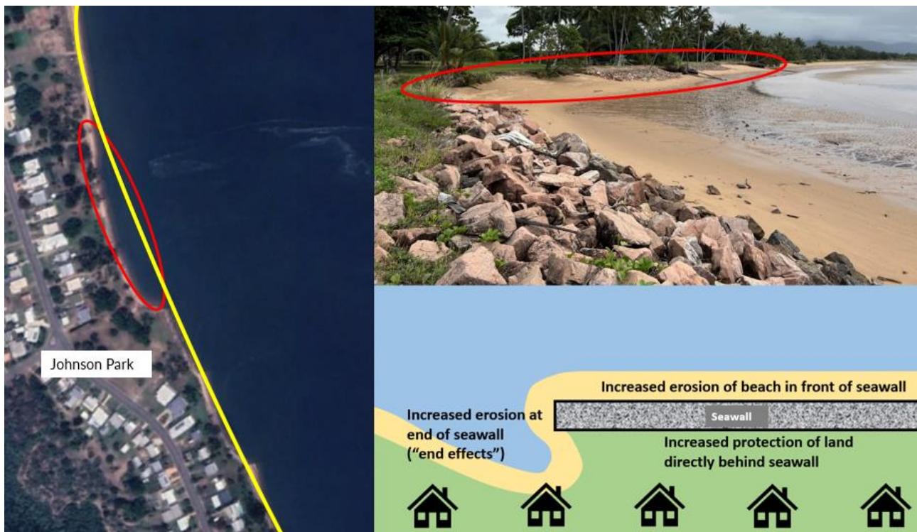
Figure 4-4 Terminal Scour Observed at the downdrift (northern) end of the Johnson Park Seawall
