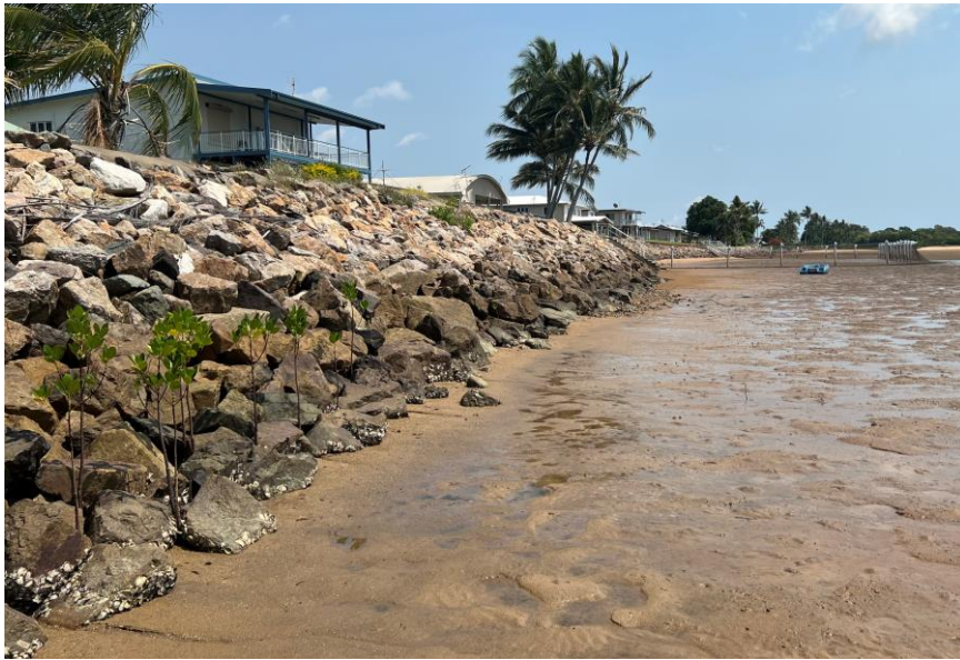
Figure 4-8 Informal rock armour seawalls at Southern Taylors Beach
